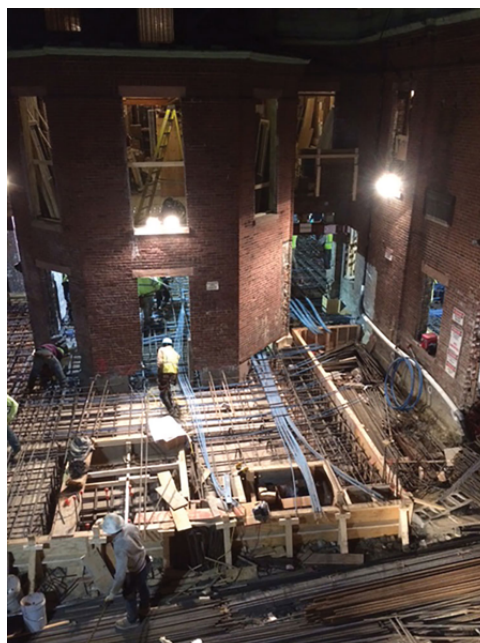
Post-tensioning tendons running through the walls.
